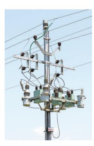
Pole mounted capacitor banks are fixed at 11 KV or 33 KV distribution network feeder. Mounting structure is made in welded galvanised M. S. angle where H. V. capacitors, capacitor switch, other accessories are mounted.
